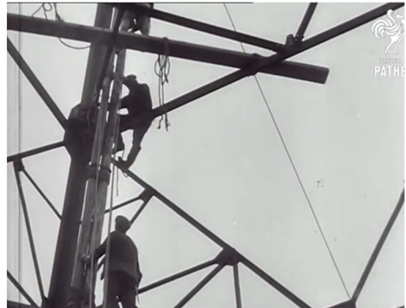
Building the tower at Alexandra Palace. Pathe News film on Youtube.
