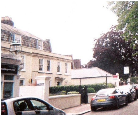
Woodside House Winchmore Hill Green
