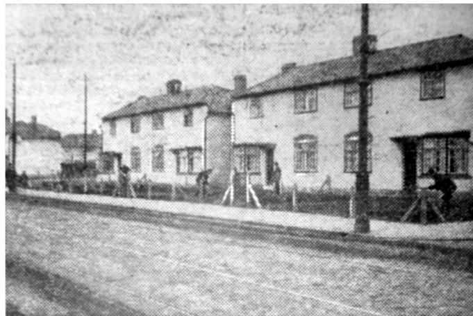
The houses in Southbury Road
