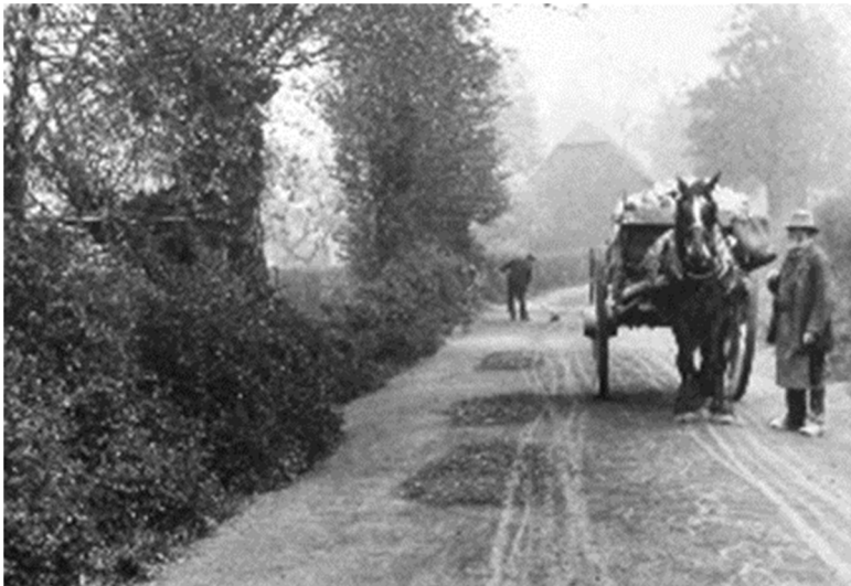
Road repairs Powys Lane 1897
